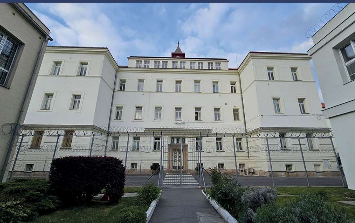
Pankrác Remand Prison and Security Detention Facility, Prague
